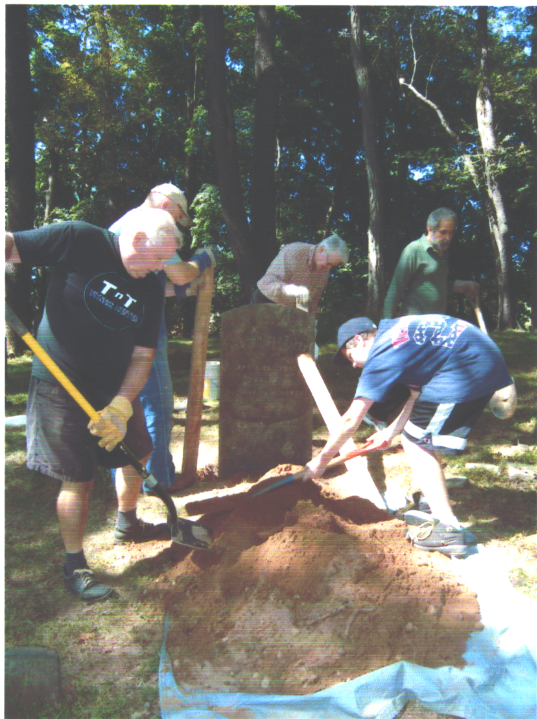
Figure 6: The team backfilling the reset stone
